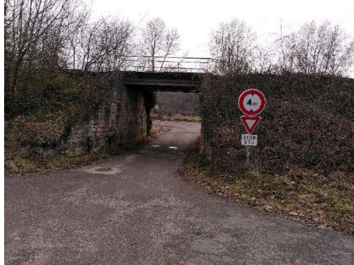
Photo 49 : Pont SNCF – Arcambal (BIEF).
